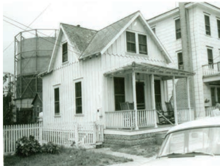
114 W. SCHELLENGER AVE. Demolished in 1974 to make way for low income housing
